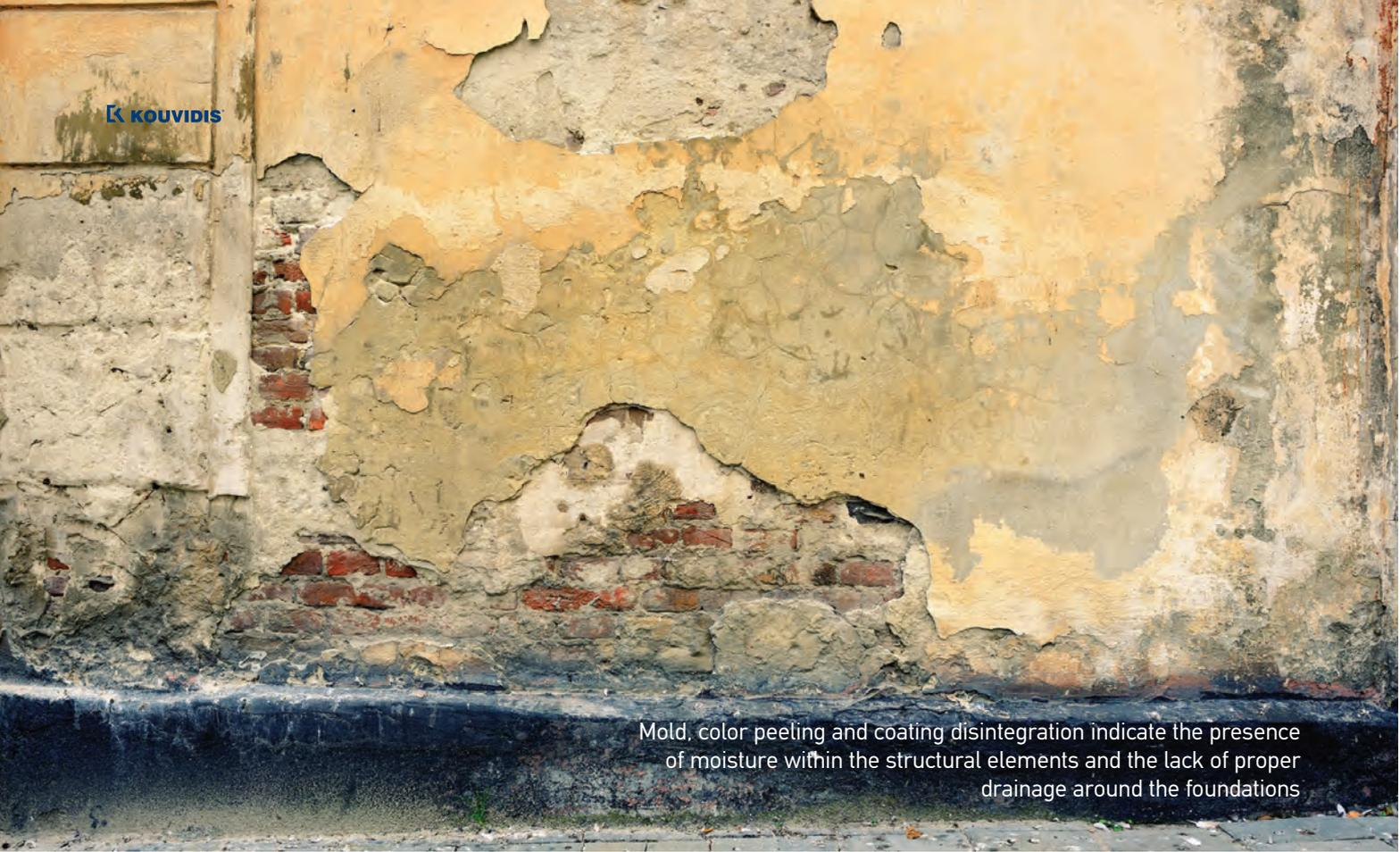
Mold, color peeling and coating disintegration indicate the presence of moisture within the structural elements and the lack of proper drainage around the foundations
